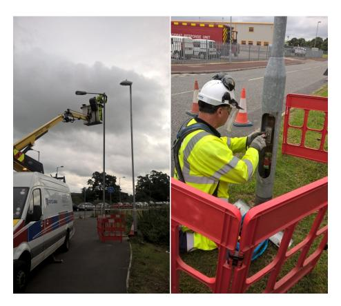
With an aging stock of street lighting a programme of both concrete and steel column testing is underway by Ringway to keep the lighting safe. A programme of removing life-expired concrete columns whilst introducing LED equipment with reduced energy consumption and maintenance requirements will continue as funds permit.
